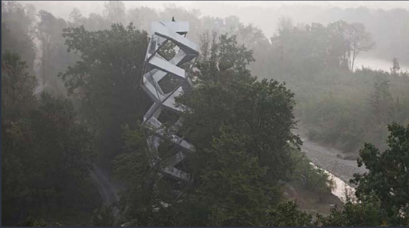
Figure 1.3 - The overall shape of the tower is based on the double helix which creates a continuous shape rising out of the canopy. The winding stairs creates a journey for the visitors to experience as they climb to the top to look out over the trees and river. The second staircase takes the visitors back down which creates another adventure back down to the ground.
