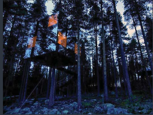
Figure 1.2 - The mirrorcube shown below is a hotel designed by Tham & Videgard. The base of the structure is aluminum and is 4 meters by 4 meters. The exterior is covered in glass to make it seem as though it is camouflaged into the forest around it. This structure is two stories and according to the booking website it can house at least two adults and a child. This treehouse is apart of a series of treehouses that are used as hotel rooms in the same forested area.
