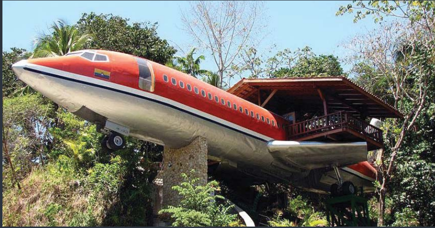
Figure 1.1 - The hotel room inside this refurbished Boeing 727 has space enough for two bedrooms. The back half of the plane rests in the trees while the front half is perched on a 50 foot tall column. The interior was refurbished with hand carved furniture and the fuselage is finished with wood siding to create a warm cozy feeling.
