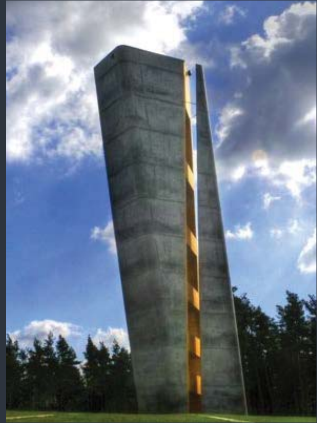
Figure 1.4 - The Arche Nebra was designed on top of a 3,600 year old solar disc. The discovery of the sky disc led to the design competition to build a structure and a tower to showcase the disc and the surrounding area. 1 Holzer Kobler designed the tower to sit exactly on top of the discovered disc and be functional. The tower leans at a 10° angle to the north and has a glass crevice the height of the tower in order to replicate the sky disc's original purpose. 1
