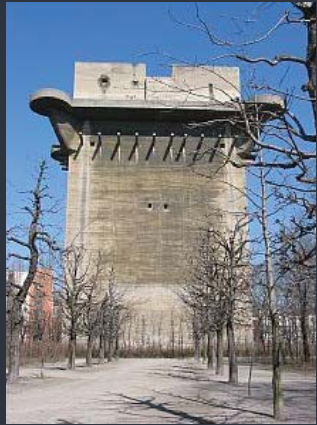
Figure 1.8 - The Hochbunker was designed and built during World War II. This blockhouse was designed to withstand bombings and air raids in order to keep the troops inside safe from the explosions. The Germans built this type of blockhouses because they were unable to build deep underground bunkers to hold large amounts of soldiers. These blockhouses were typically built out of concrete.
