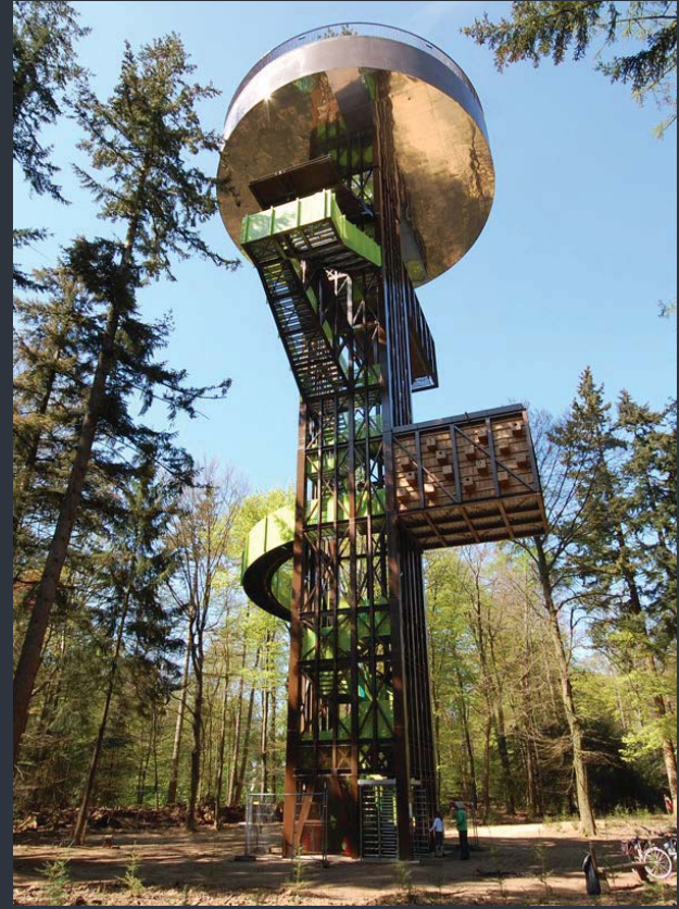
Figure 2.8 - The perspective shows all of the different lookouts on the tower from the lowest enclosed box lookout to the mirror ceiling lookout nearly at the top to the disc at the very top. Also it shows the arcing ramp on the side along with the protruding stairs near the top.
