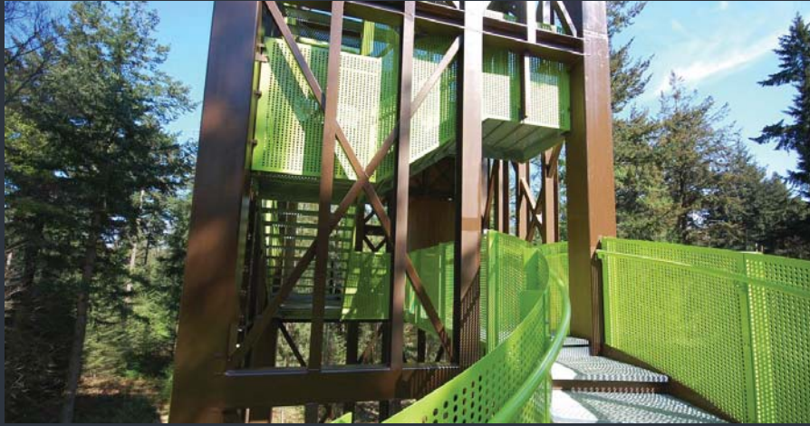
Figure 2.7 - The stair ramp protrudes out the side of the tower and wraps around and re-enters at the floor for the first lookout point along the journey upwards. This ramp really changes the shape of the tower because the ramp and the top disc are the only circular shapes in the whole tower. The rest of the tower is all based around squares and rectangles.
