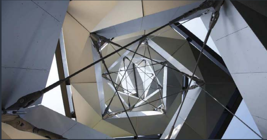
Figure 2.1 - This image shows what looking up into the tower from the base looks like with the double helix stairs. The twisting stairs are held in place with large steel members that following the shape on the exterior of the stairs while the interior is held in place with smaller steel straps for lateral bracing.
