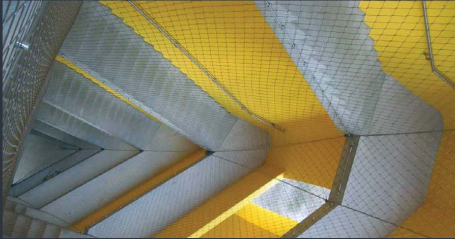
Figure 2.19 - An interior perspective showing the stairs as they wrap around the interior of the tower along with the windows that open into the crevice. By placing now railing on the inner portion of the stairs it creates a clean look all the way up and out of the tower.
