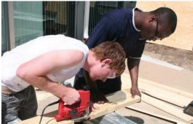
Figure 4: Project 2 Build Day – Left the Groups in Various States of Construction; Right N. Bosman and D. Ojo Cut a Birdsmouth Notch.
