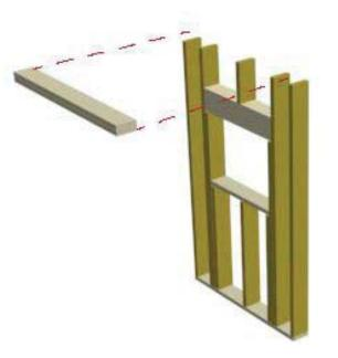
3j) Place first 4' 2x6 member on top of studs and nail down, then repeat for the second top plate.
